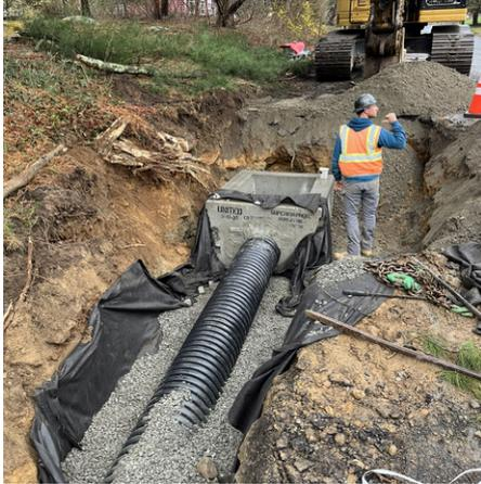
Work continues to progress along Botsford and Bungay Road. The contractor has completed tree removals to make way for upcoming sidewalk and retaining wall installations. In addition, new catch basin tops and drainage pipes have been installed along Botsford Rd. These upgrades will improve drainage in the area, helping to protect the road's overall integrity and ensure its long-term durability.
